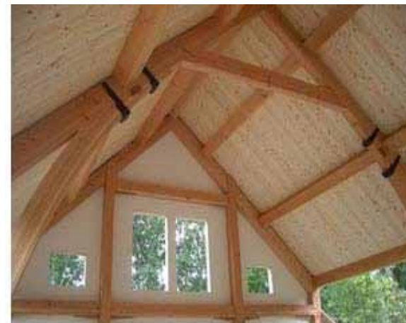
Fig. 36 typical Bensonwood heavy timber framing
