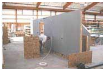
Fig. 34 preassembly of an interior wall
