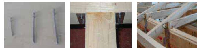
Fig. 11 the double-headed nail in conjunction with metal hangers and plates creates a system that is more easily disassembled than traditional construction techniques
