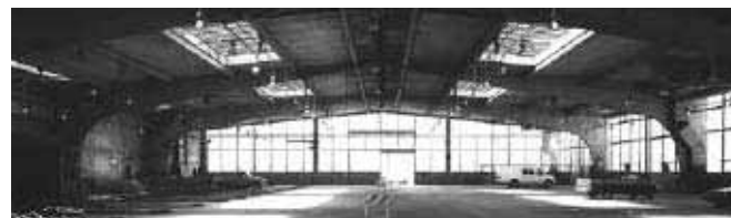
Fig. 47 The 1951 SOM bus maintenance facility required seismic bracing, toxic soils remediation, and other treatments. Photo: Richard Barnes
