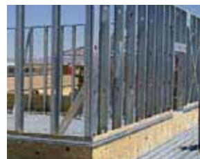
Fig. 73 light-gauge metal framing
