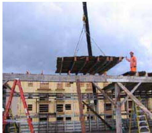
Fig. 13 panelization of roof structure
