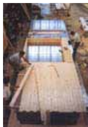
Fig. 28 off-site construction of panels
