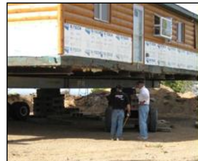
Level III Alteration Example – Repositioning a Building
