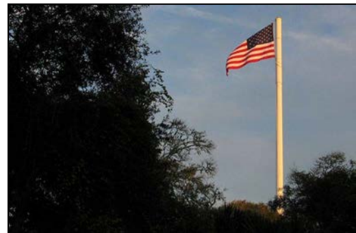
Wireless Tower Camouflaged as Flagpole
