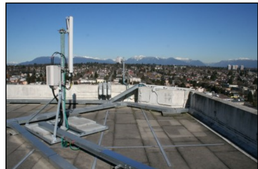
Antenna Attached to Roof of Existing Building
