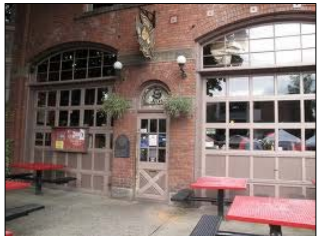
E-9 Restaurant, an example of a TI conversion from a fire station to a restaurant use.
