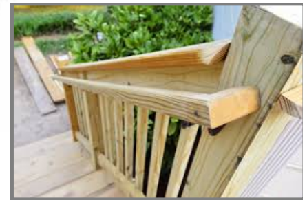
Stairs with guardrail and a handrail
